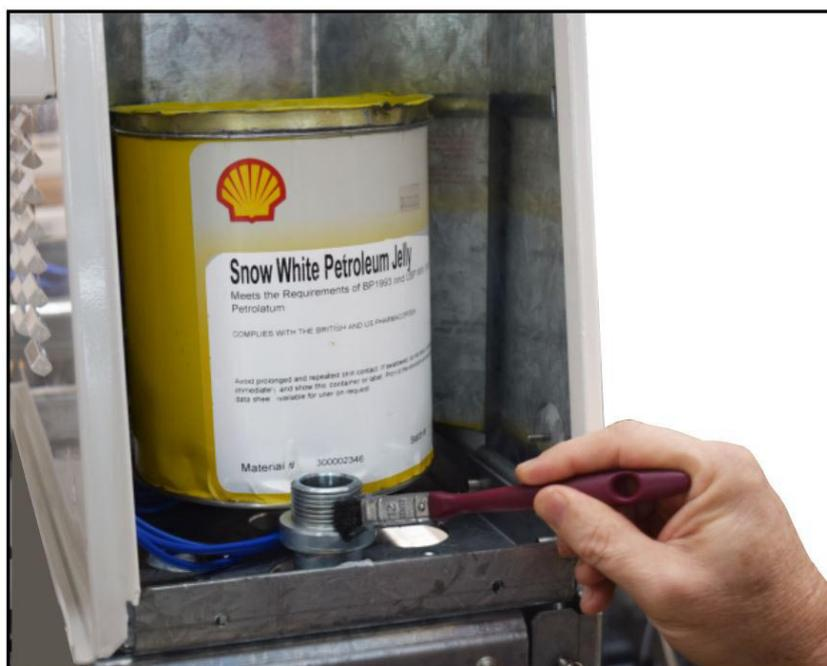
Figure 1. Greasing Threaded Connections
