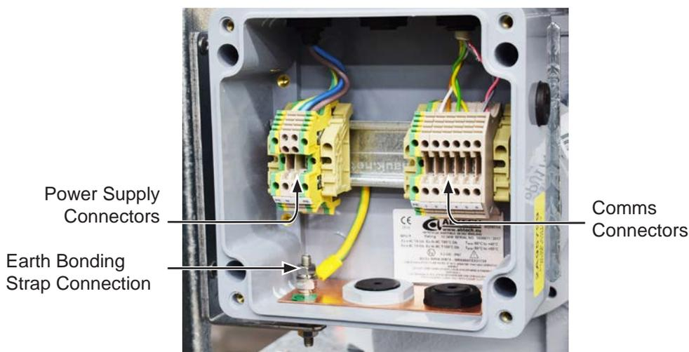
**Figure 7. Single Phase Pump Connector Blocks**
