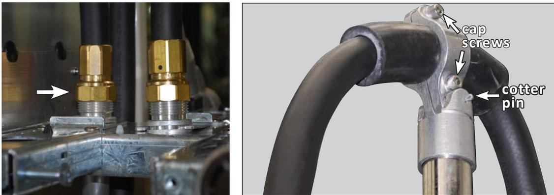
**Figure 29. Brass Swivel Nuts and Hose Clamp**
