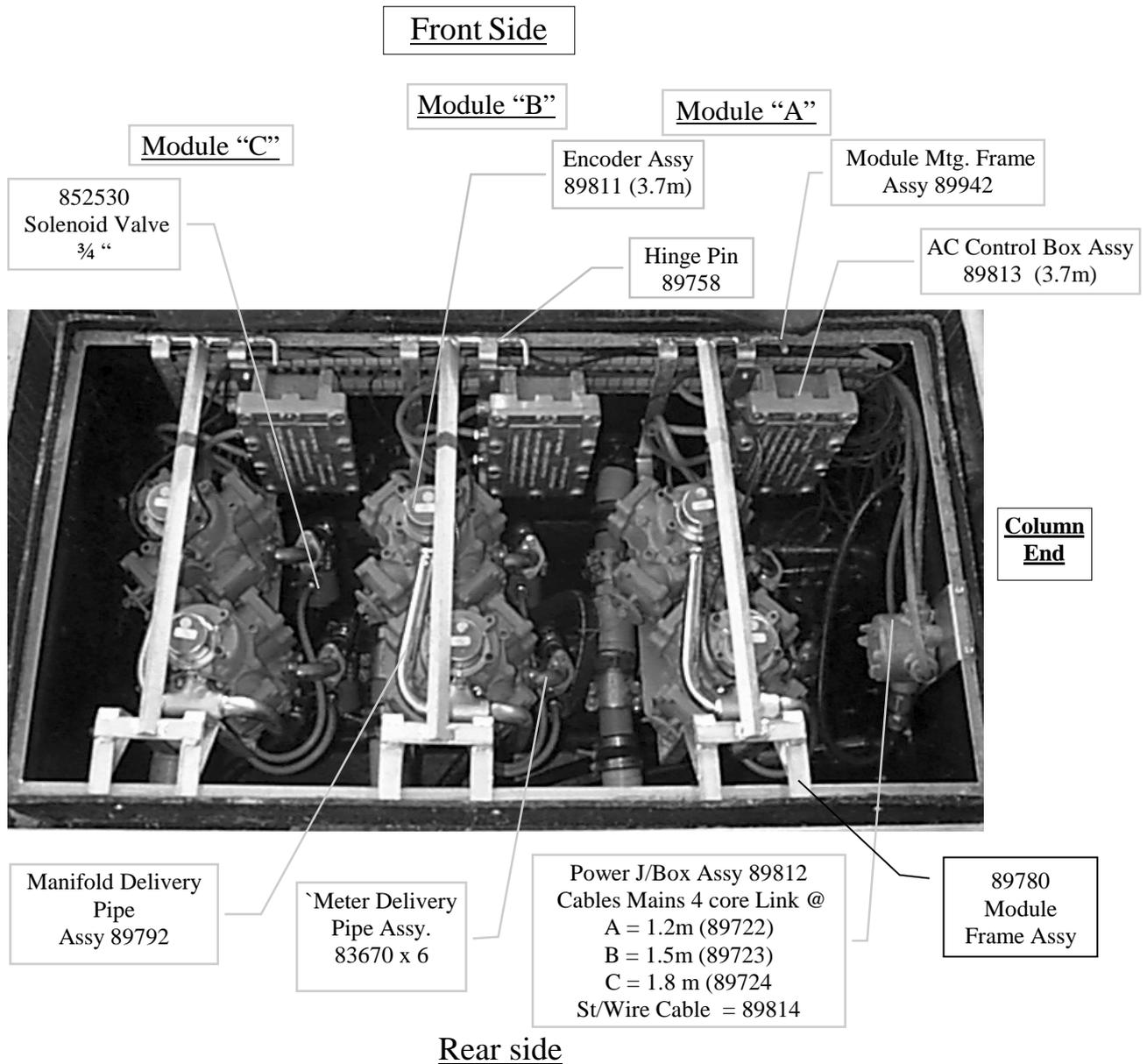
Produce Feed Hose Assy - 3/4 in Hose - 3/4 Female/Female Sw/nut - 1.050 m 3/4 (Feed Line to Module) x 3
